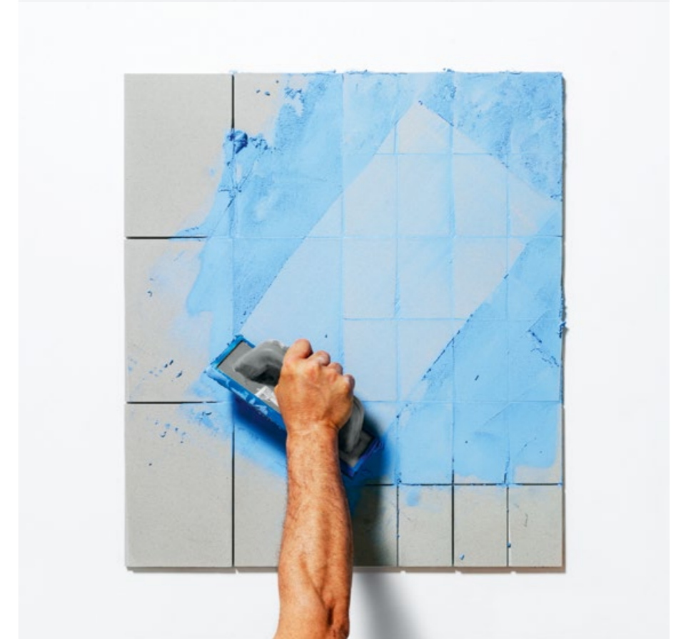
posa e stuccatura / laying and grouting formato / size: large + small
